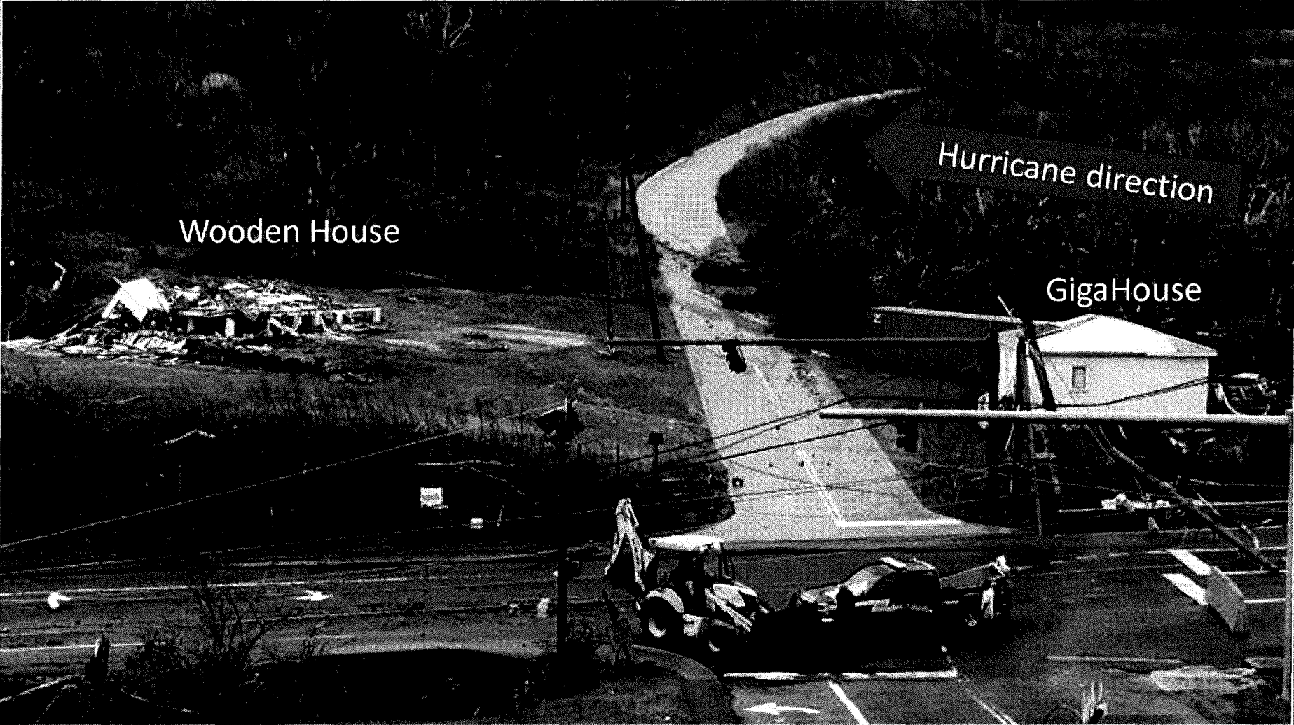
St Thomas USVI GigaCrete Caribbean Sales Office after Hurricane Irma and Maria, note the stripped trees everywhere and the wood framed building across the street, completely destroyed.
