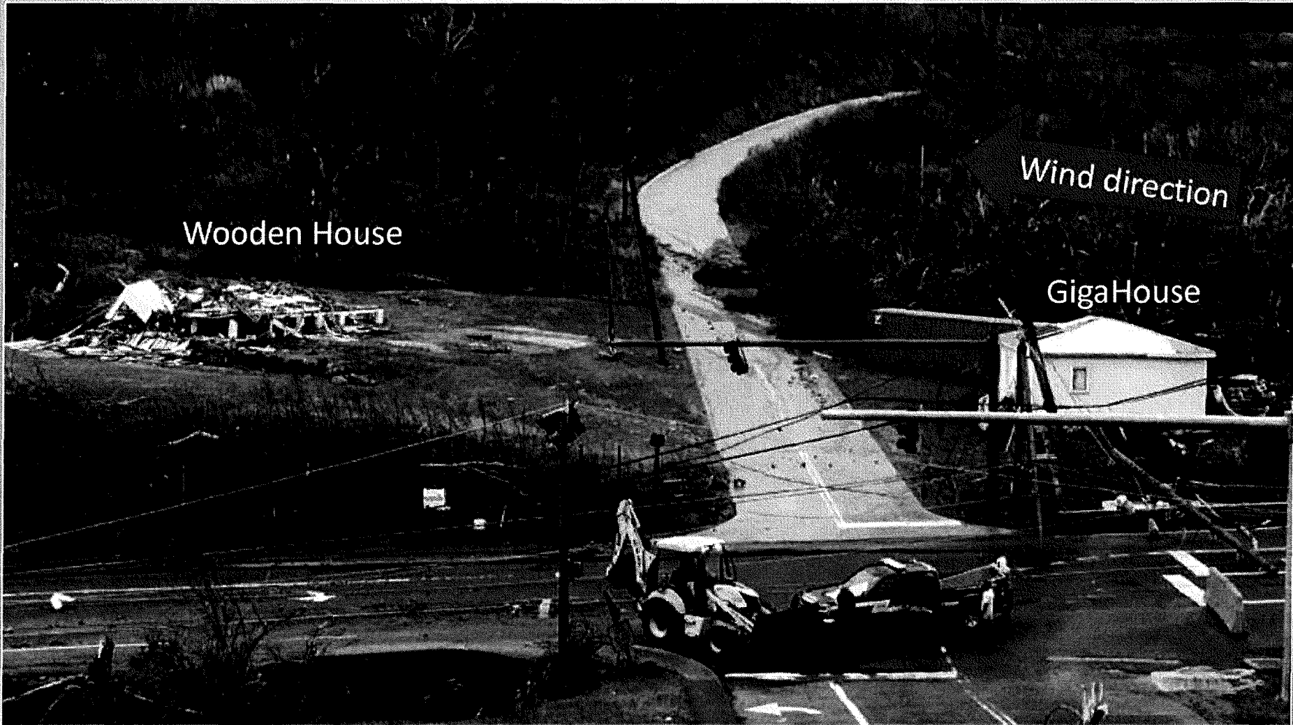
St Thomas USVI GigaCrete Caribbean Sales Office after Hurricane Irma and Maria, note the stripped trees everywhere and the wood framed building across the street, completely destroyed.
